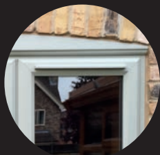
Trickle vent through a Rebated Sash
